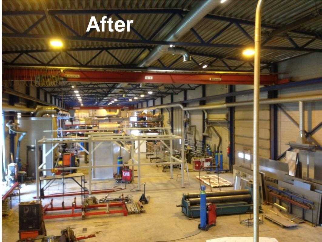
A welding shop was renovated by installing a new ventilation system which included heat recovery and hybrid air distribution systems. After the renovation, the workers exposure to contaminants was reduced significantly. The improved air quality is clearly evident in the following chart results.
